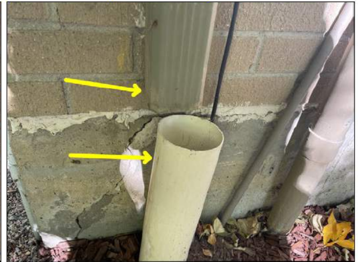
Reconnect downspout with the drain southwest corner of the house
