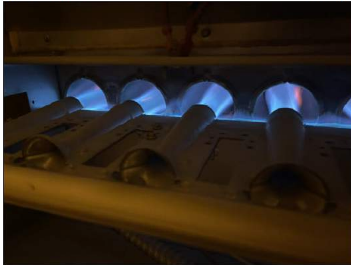
Furnace burn chamber
