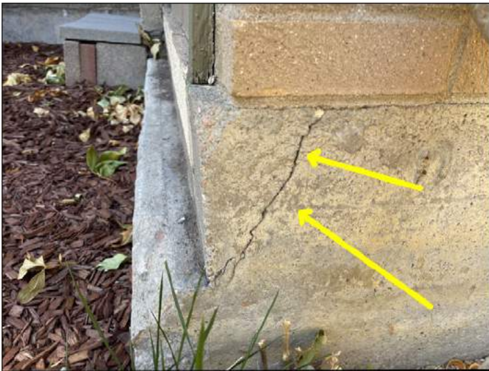
Monitor minor crack on the south east corner
