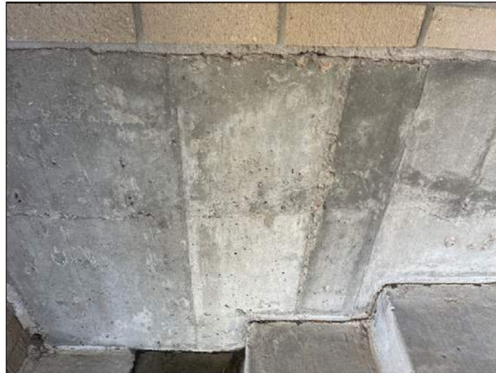
Minor crack southwest corner of the home
