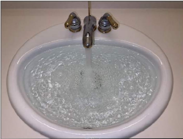
The sink is filled to test the drain connection
