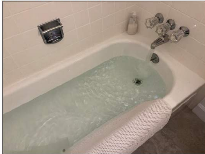
The bathtub is filled to test the drain connection
