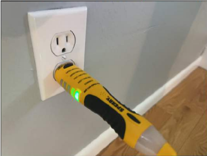
Outlet on the North wall of the north east guest bedroom has correct copalum wiring
