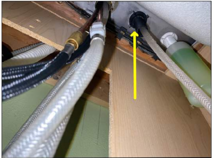
Connection to the sprayer is leaking
