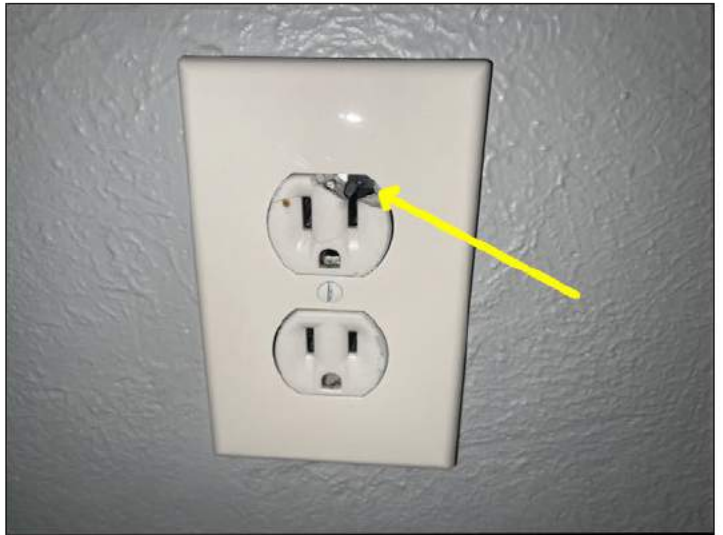
Broken plug south wall in the family room
