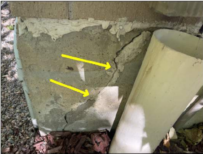
Minor crack southwest corner of the home
