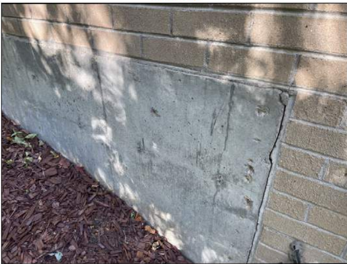
Monitor minor crack on the south east corner
