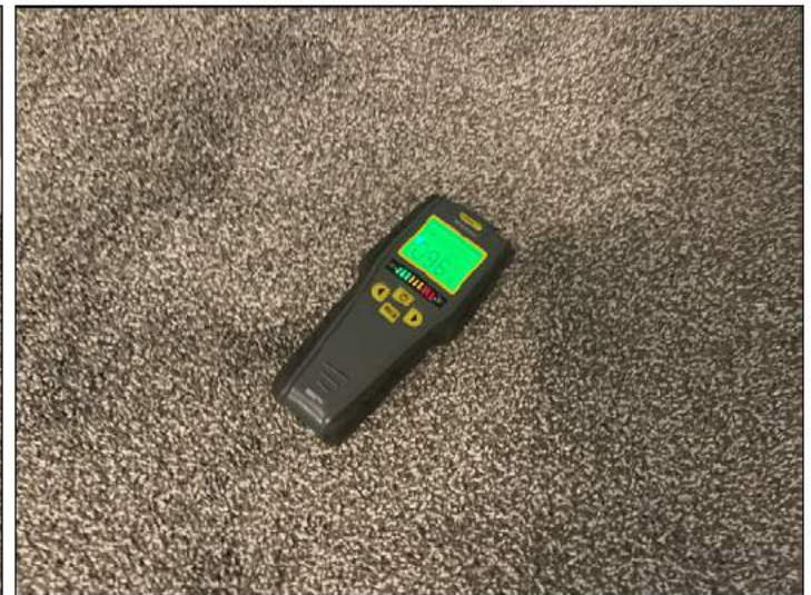
Moisture meter showing wet carpet in the basement
