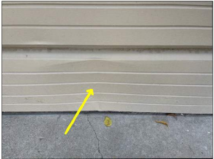
Minor dent in the west garage door
