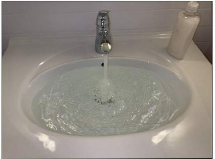
Sink is filled to test the drain connection
