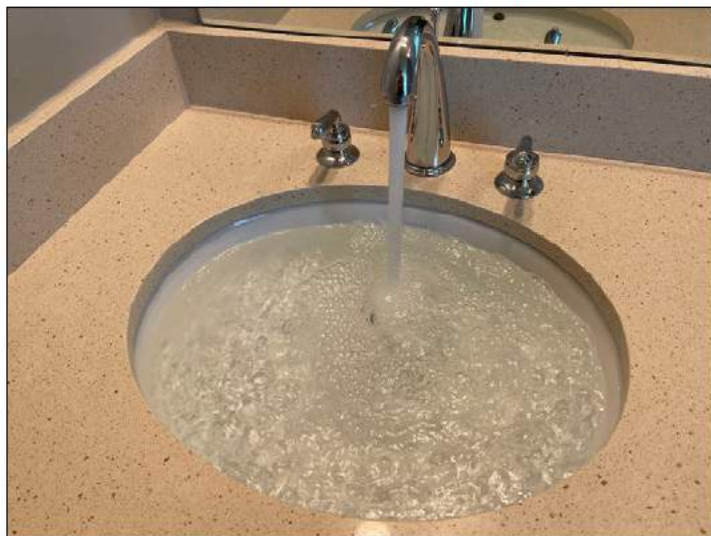
Sink is filled to test the connection
