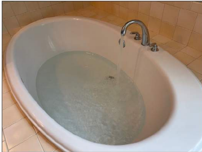
Bathtub is filled to test the drain connection
