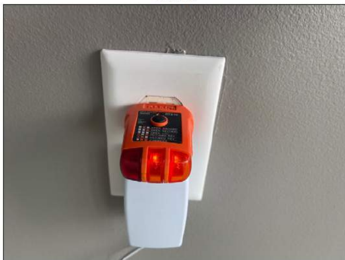
Outlet with reverse polarity north wall of the office
