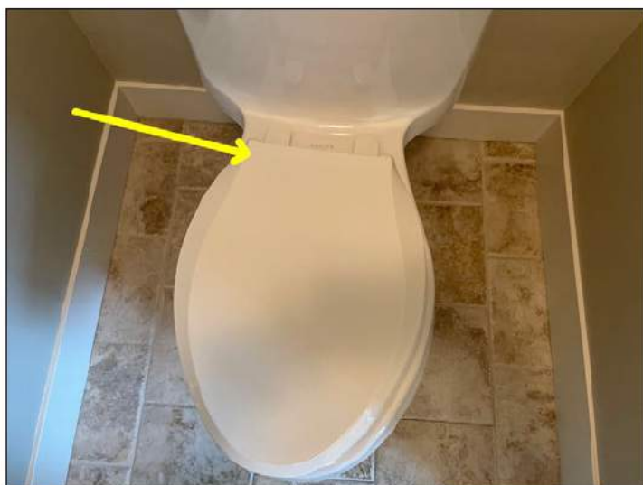
Seat is loose on one side
