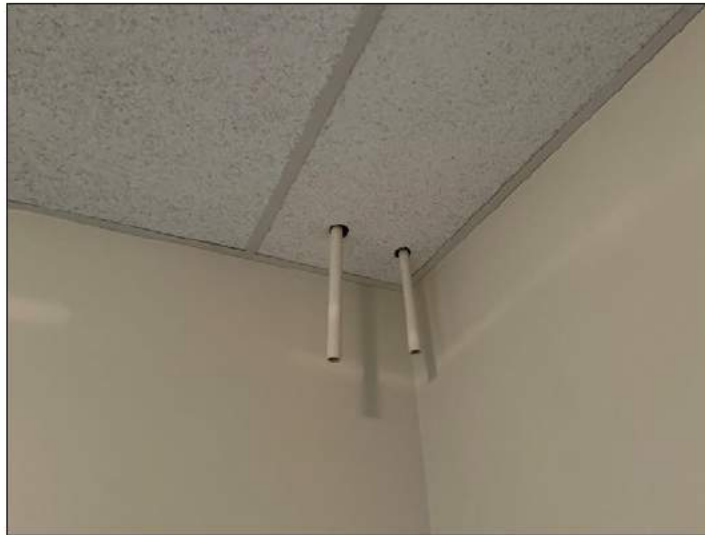
Condensation tray for both Fan Coil systems drain here
