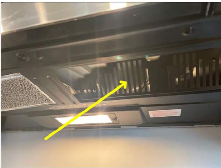
Missing a filter/vent cover
