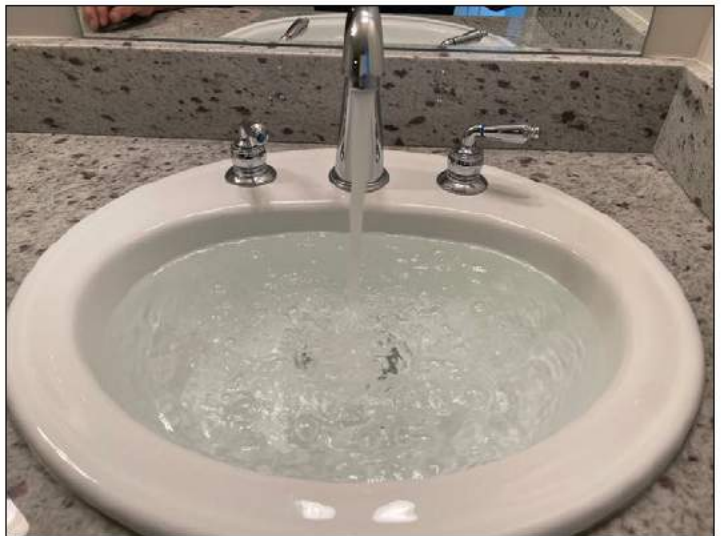
Sink is filled to test drain connection
