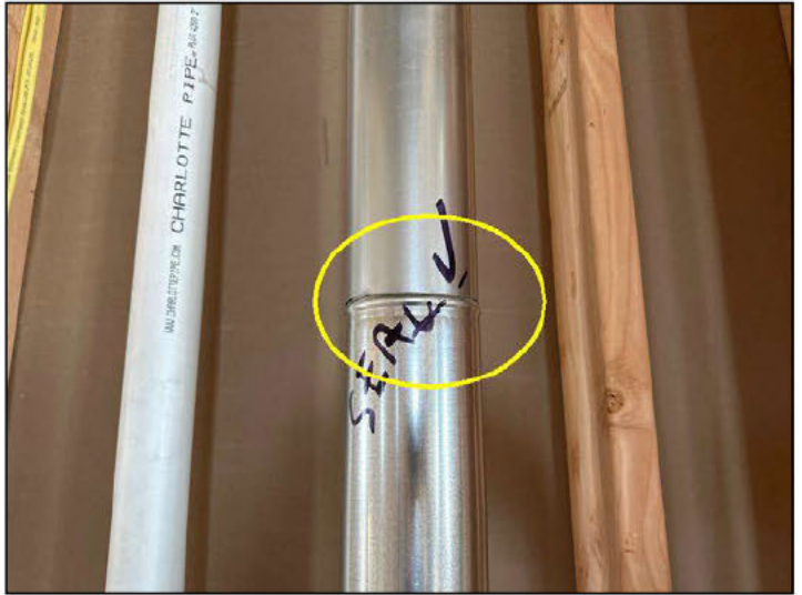
Seal seam at the dryer vent
