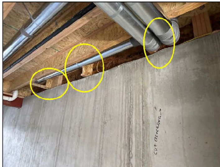
East wall tinner cut out blocking
