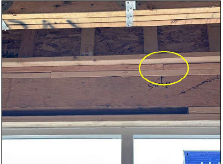
Missing strap at plate break east wall above primary bedroom window
