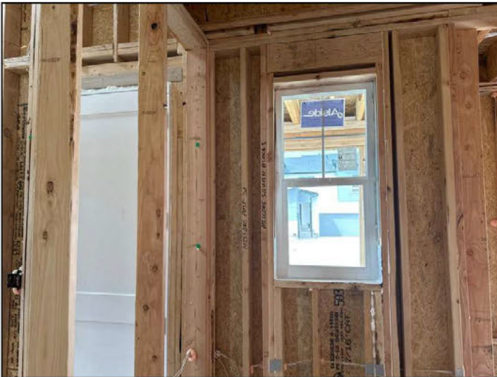
Missing squash blocks and post west wall office south of the window
