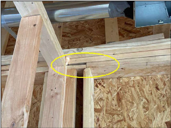
Strap needed at plate break north-west corner primary toilet
