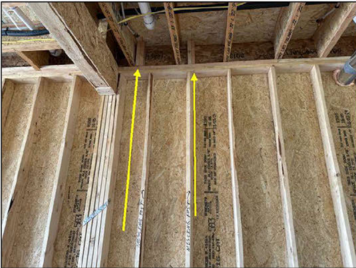
Missing posts for squash blocks north wall garage east of the I beam
