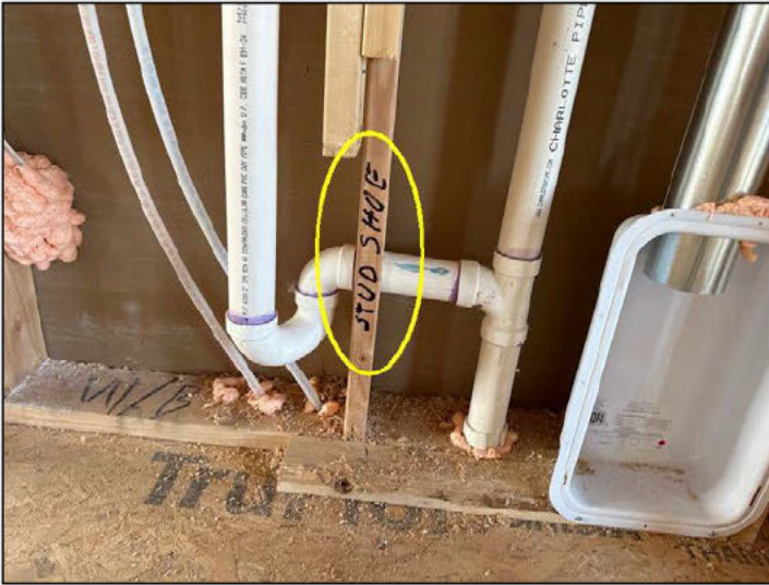
Missing stud shoe at plumbing south wall laundry
