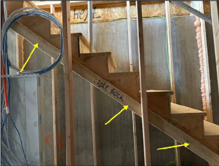
Missing fire block at the stair stringer both sides
