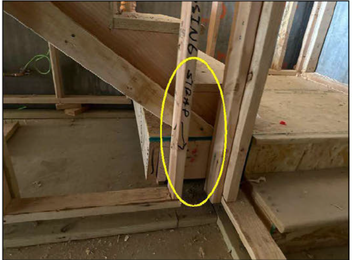
Basement stair landing not strapped
