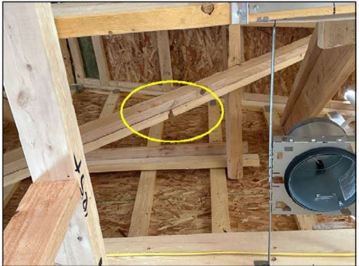
Second truss in from the north is broken with improper fix from the framer
