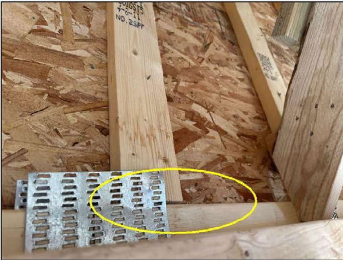
West end gable gusset plate not covering truss member
