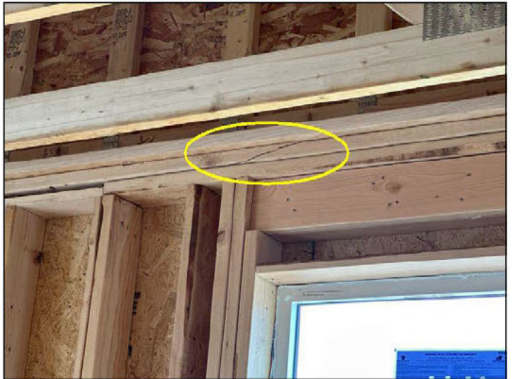
Missing plate break strap top of the south balloon wall west of fireplace
