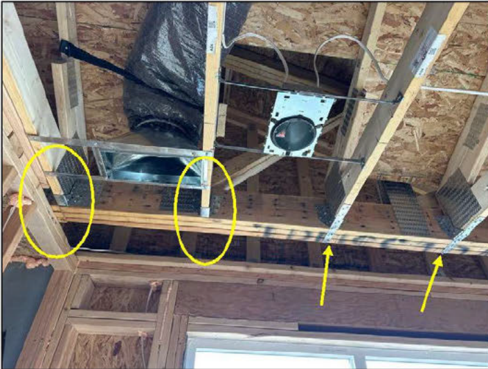
Missing straps near east window primary bedroom truss to girder
