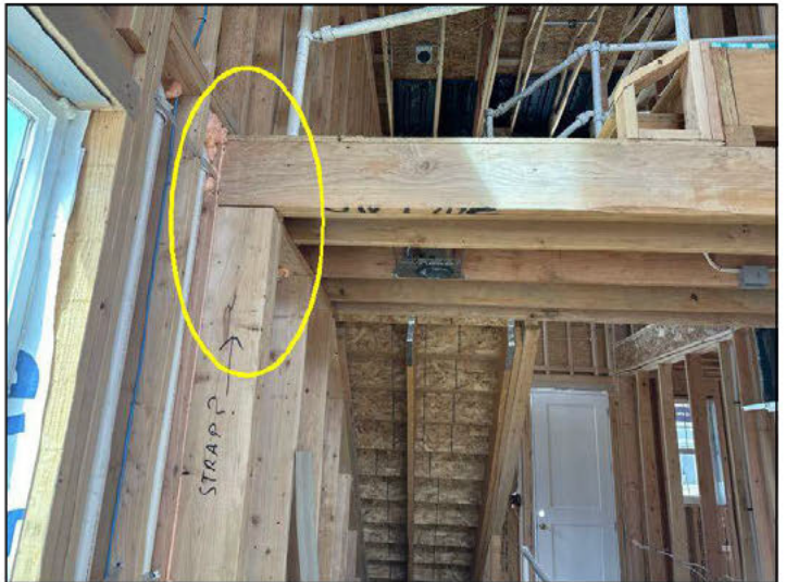
Missing strap west wall near south exterior wall stair landing
