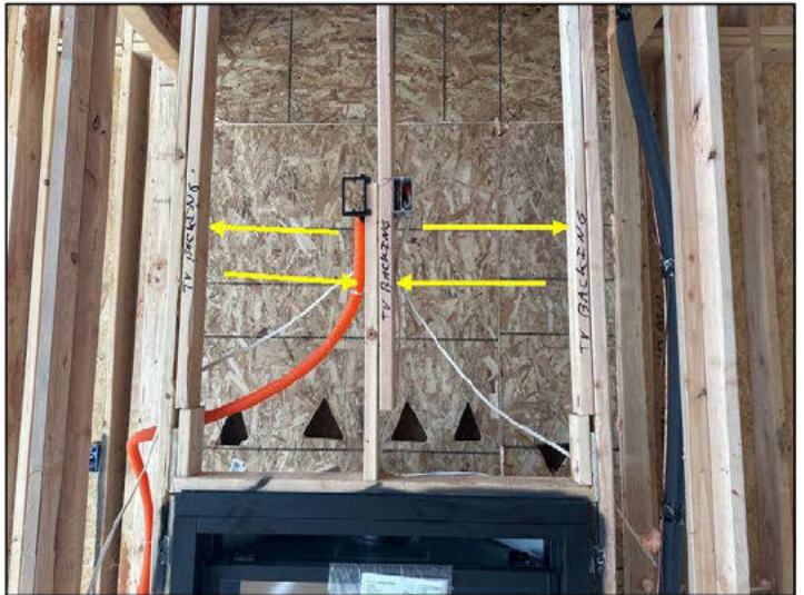
Add backing for TV south wall above the fireplace
