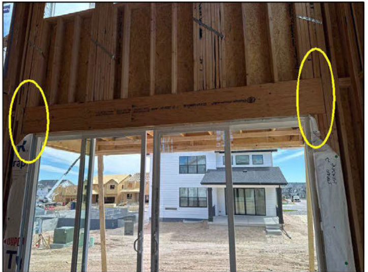
Strap headed over the sliding glass door
