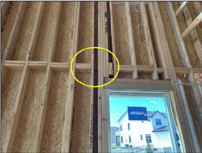
Missing 10' fire block south wall west of fireplace
