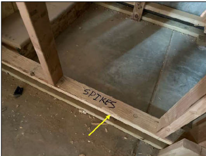
Missing spikes in the floating wall
