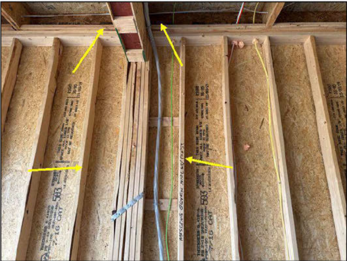
Missing squash blocks/post north wall west of the I beam
