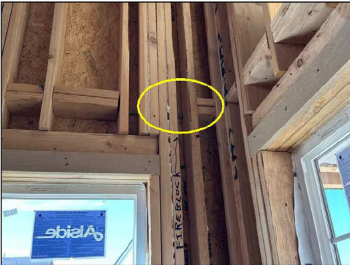
Missing 10' fire block south-west corner above the stair landing
