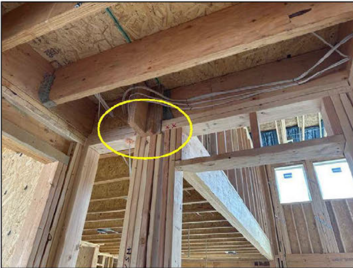
Cut LVL flush east wall mud room
