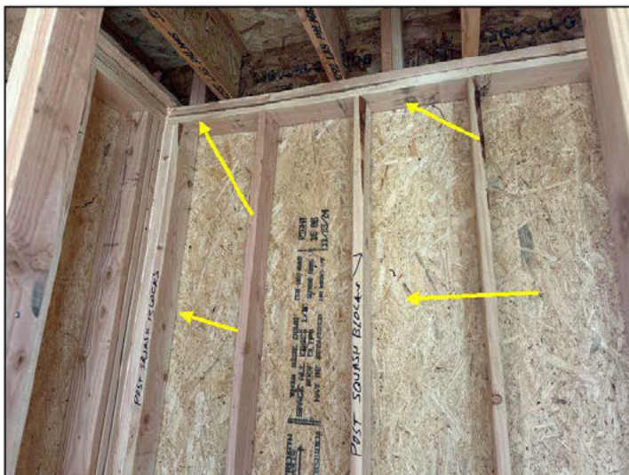
Post squash blocks north wall in pantry
