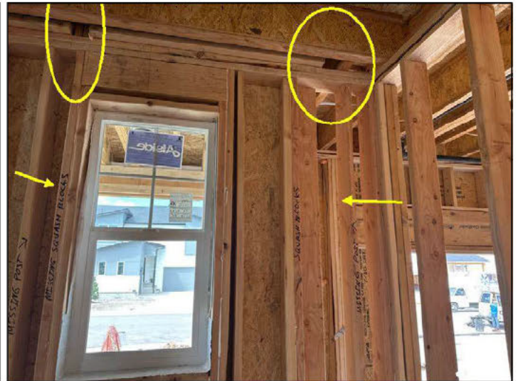
Missing squash blocks and post west wall office north of the window
