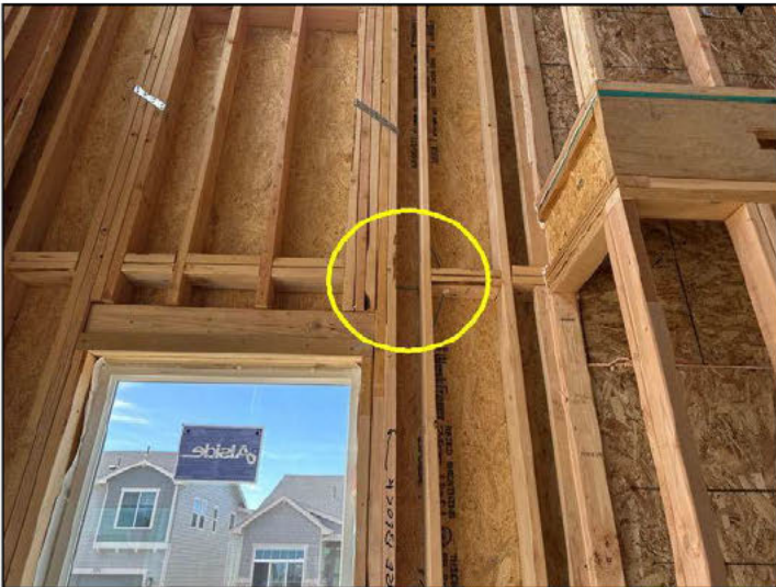
Missing 10' fire block living room south wall east of fireplace
