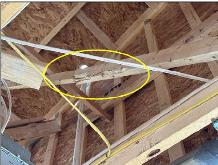
Second truss in from the north had a broken web 2x4
