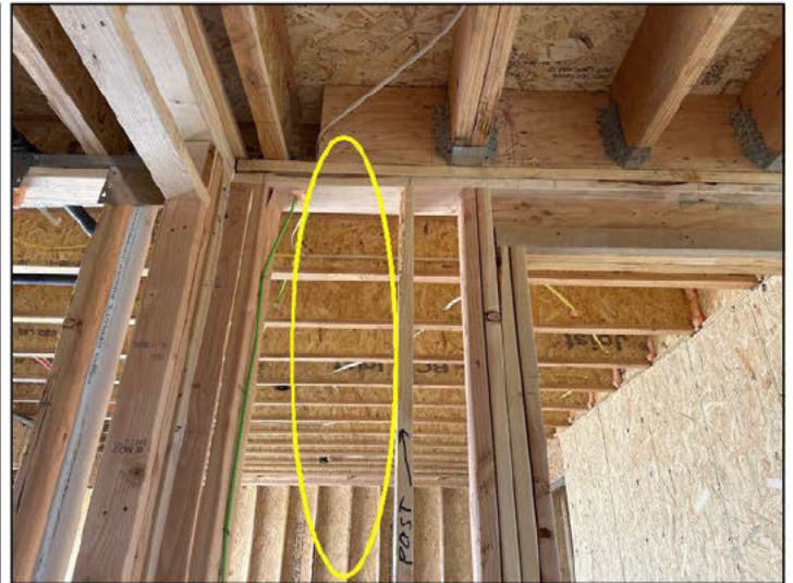
Missing post north wall mud room west of garage occupant door
