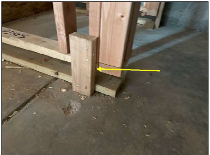
Remove temp blocks after spikes are in
