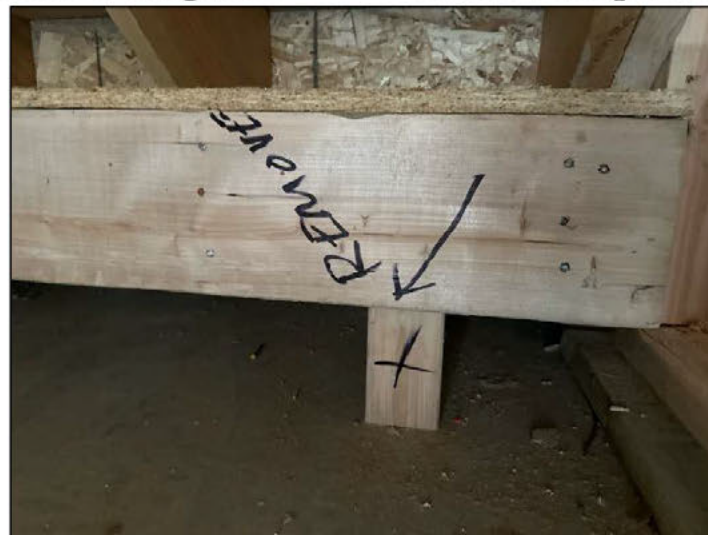
Remove temp block under the west end of the basement stair landing after straps are added
